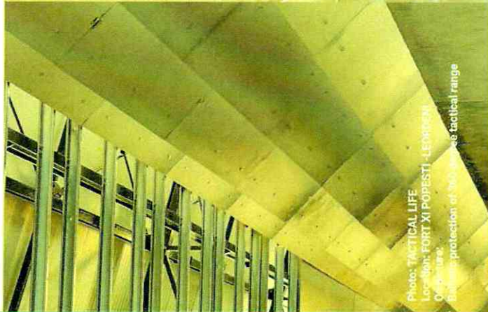
Photo: TACTICAL LIFE Location: FORT XI POPESTI - LEONARD On picture: Ballistic protection of 380 degree tactical range
